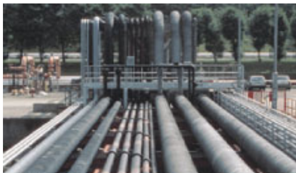
● Pipe laying in pier
