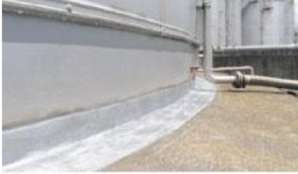
● Around a tank base (to prevent rain water penetration)
