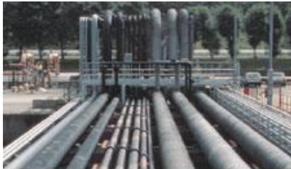
● Pipe laying in pier
